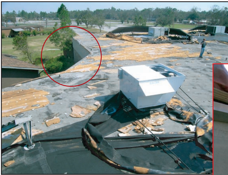
Figure 2: Deformation of light gauge cleats in strong winds can allow roof edge metal to bend upward and begin peel of fully adhered roof membranes (excerpt from Phil Dregger presentation).
