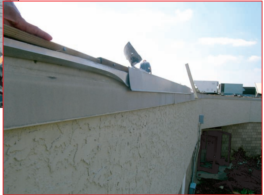
Figure 2: Deformation of light gauge cleats in strong winds can allow roof edge metal to bend upward and begin peel of fully adhered roof membranes (excerpt from Phil Dregger presentation).
