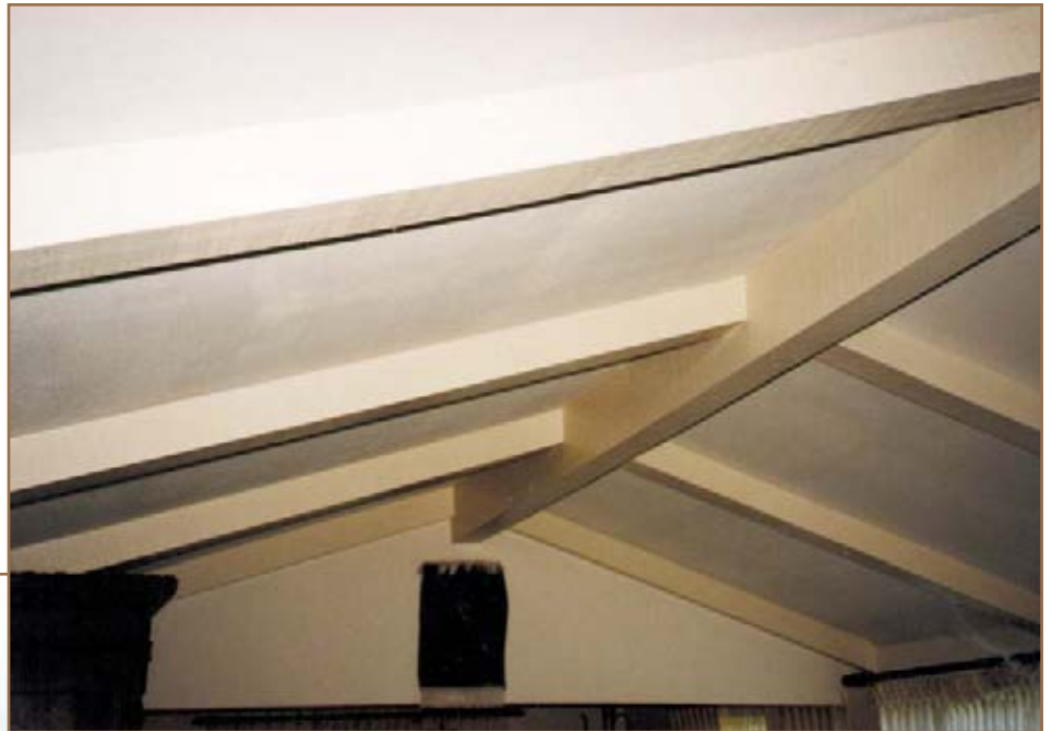
Photos 1 (left) and 2 (above) - Steep roofs without conventional attic spaces (e.g., enclosed rafter spaces).
