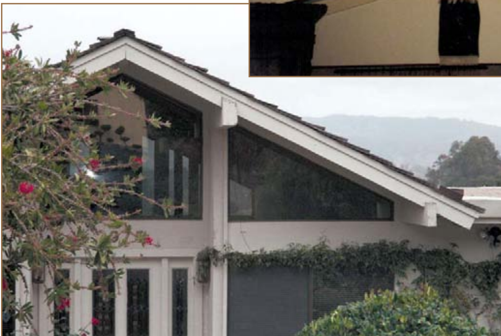
Photos 1 (left) and 2 (above) - Steep roofs without conventional attic spaces (e.g., enclosed rafter spaces).
